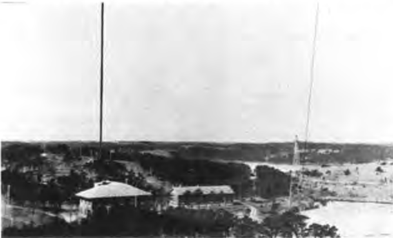
"Hotel DeGink" - and the Operating Station of "WCC" at Chatham, Mass
